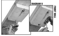
Mount **2" x 6"** x 7" (50 mm x 152 mm x 180 mm) riser board on front mounting board centered between the two pigtail lag screws (B). Drill  $\frac{5}{32}$ " (4 mm) holes. **Always wear safety glasses.** Attach riser boards using two  $\frac{1}{4}$ " (6 mm) lag bolts (I) and washers (J) (included). Do not overtighten.
