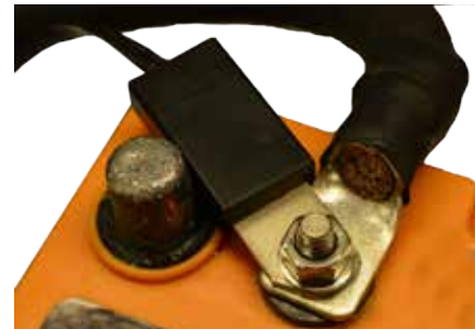
Fig 2.5(b) Temperature Sensor Installation
